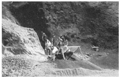
Figure 2: Volcanic ash pozzolana being excavated, Rwanda.
