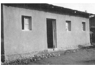
Figure 1: house plastered with lime-pozzolana mix, Rwanda.
